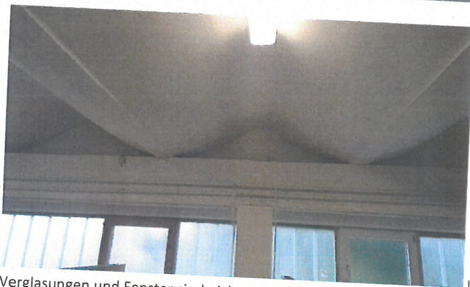
Halle, Blick in Nord-West-Ecke
